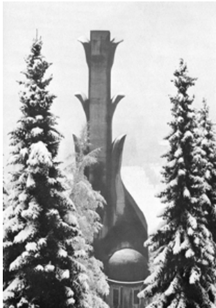
Rudolf Steiner, 'Heizhaus' (1928)
